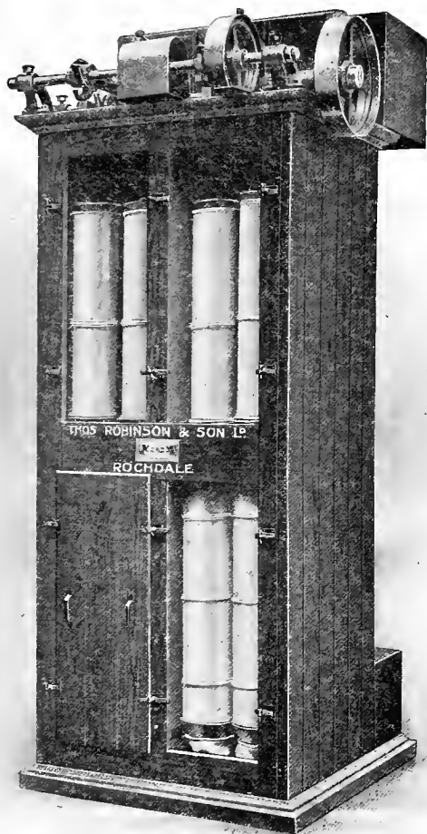
ROBINSON'S SLEEVE FILTER DUST COLLECTOR
